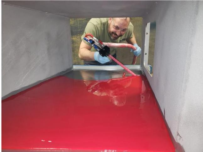
This liner can be spray applied by an SFLP spray machine, cartridge sprayer or be casted similar to that of concrete and finally the liner can be trowel repaired.
